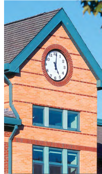
Clinton Elementary School Dedham, MA (Dore + Whittier Architects)
